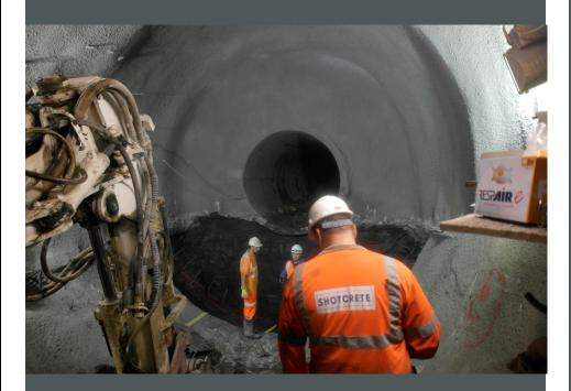
Supply and labour plant and materials to excavate and construct sprayed concrete enlargements within existing 2.85m ID tunnel.
